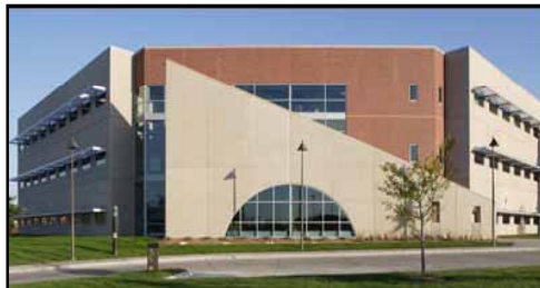
Scott Technology Center (STC)
